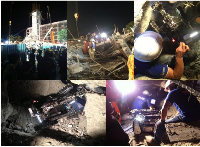
Fig. 14. On-site experienced at U-place condo, Pathumthani, THAILAND
