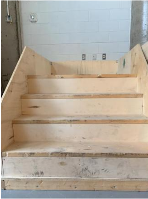
Fig. 2. Field used for testing Markhor's abilities
